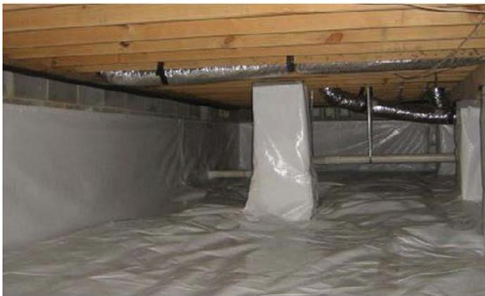
**NOTE:** Completely sealed crawlspaces (no exterior cross-ventilation) require a dehumidification system as part of the sealed crawlspace design.
